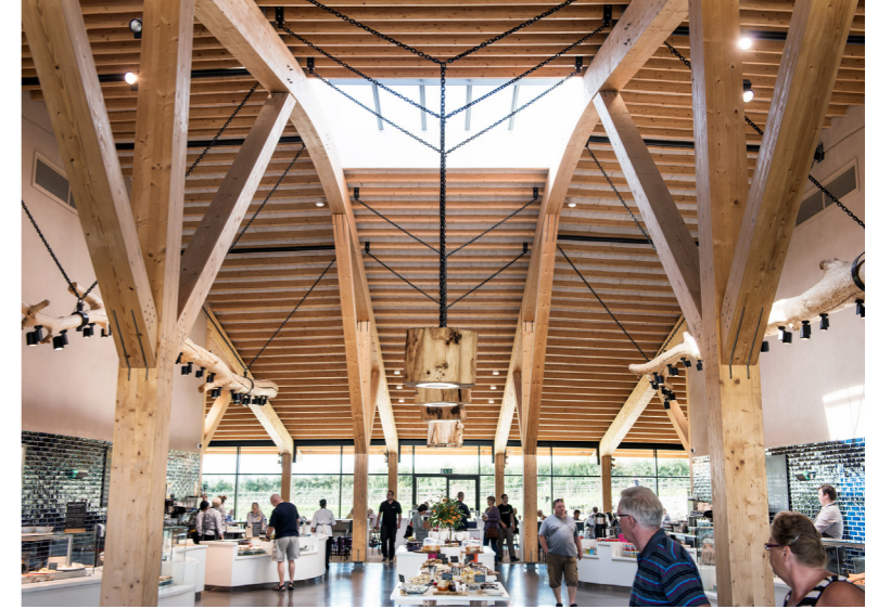
↑ Gloucester Services, Northbound, M5
